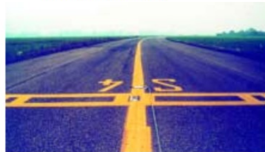
Photograph 9 - S4 marking and ICAO pattern B runway - holding.
